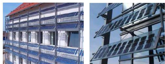
Fig 10: Outrigger PV Shading & Glass Louver System
