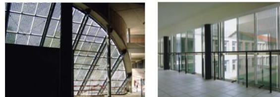
Fig 9: BIPV Transparent facade Aalst, Belgium & Semi-transparent facade a-Si.
