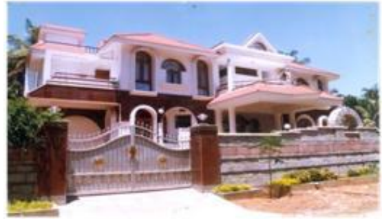
Figure 2 Shading by balcony projection in Chennai (Architect Dr.S.Ramesh)
