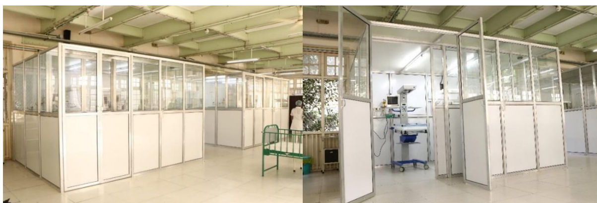
Figure 3: Installed isolation facility in hospital
