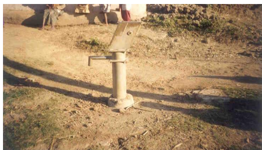
Dismantled hand pump
