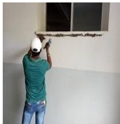
Horizontal crack
