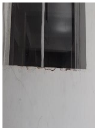
Horizontal crack
