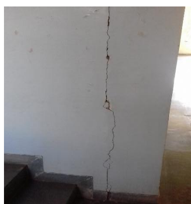
Vertical crack
