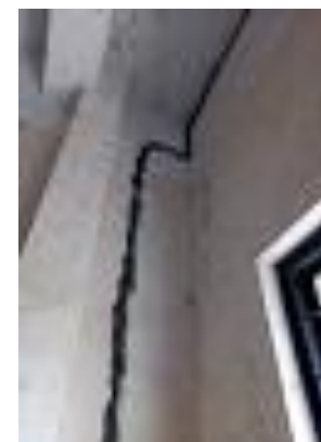
Diagonal crack
