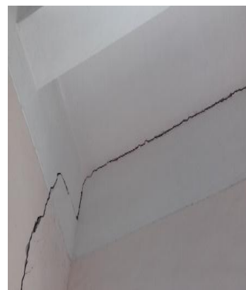
Diagonal crack
