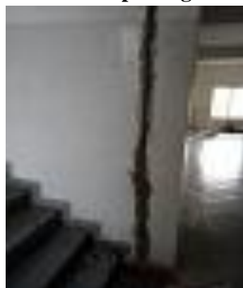
Vertical crack
